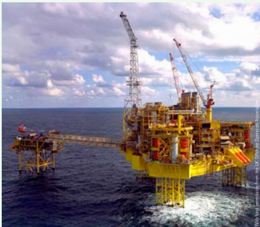
The Elgin Platform is one of the most advanced in the world. The jack-up design means that, unlike older rigs with concrete bases, it could eventually be lifted from the sea floor and reused elsewhere.
